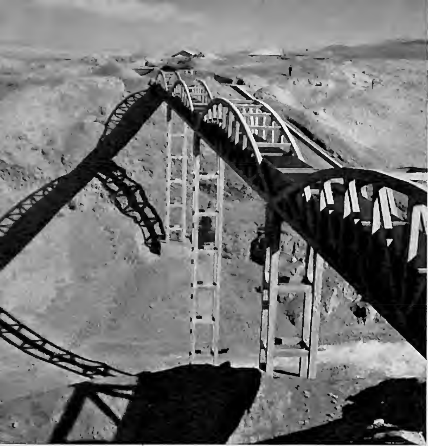
An aqueduct 92 metres long, part of the irrigation project being constructed in Tungteh County, Hainan Tibetan Autonomous Chou, to transform the Meilitan grassland.
